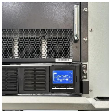
Legrand TRIMOD HE 20kVA/20kW UPS , TRI-HE-20 . Modular ...
