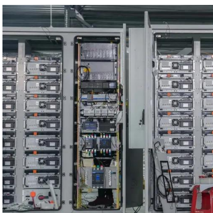
GVSCBC10B2 Schneider Classic Battery Cabinet
