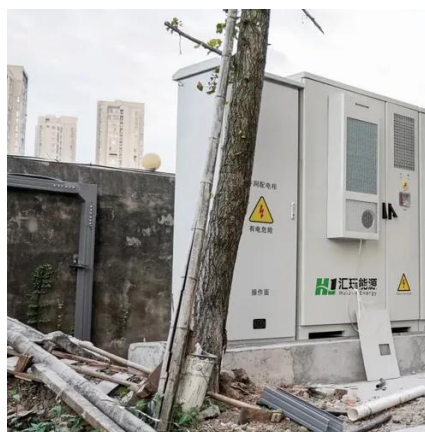
Djibouti solar battery storage solutions
