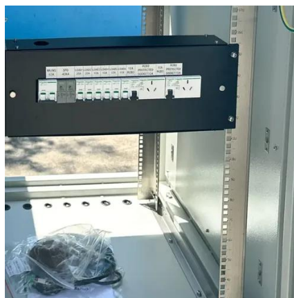
lead acid battery cabinet
