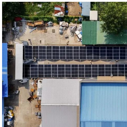
Large-Scale energy storage , Microgreen.ca
