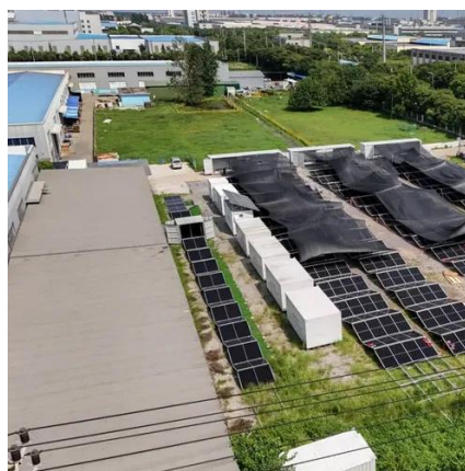
Current Transformer Cabinet On Erickson Electrical Equipment Co.
