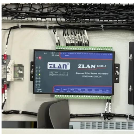
a High-Voltage Outdoor Energy Storage Cabinet of ...
