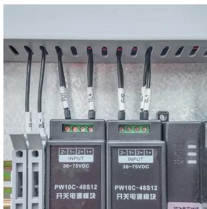
Scalable 208V Commercial BESS (20-480+ kWh)
