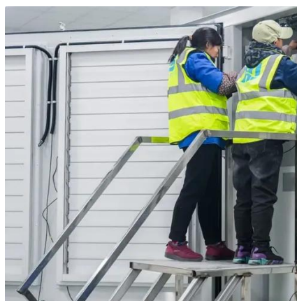
What is a solar photovoltaic grid-connected cabinet?
