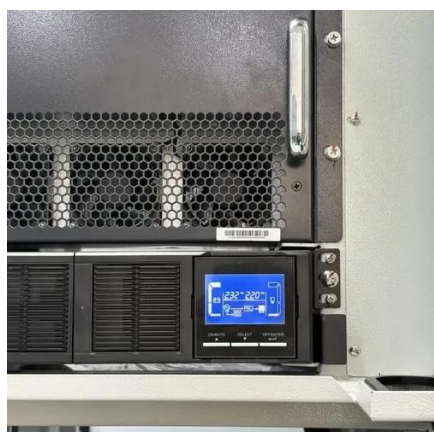
24 kW Telecom Power Cabinet with Rectifier & Distribution System
