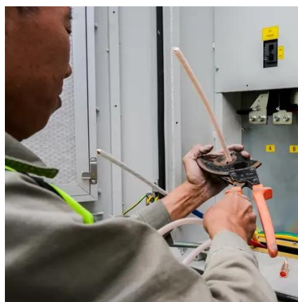
Estonia battery energy storage cabinet manufacturers ranking
